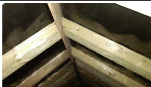
Figure 9. Modern BRM fitted to roof.
