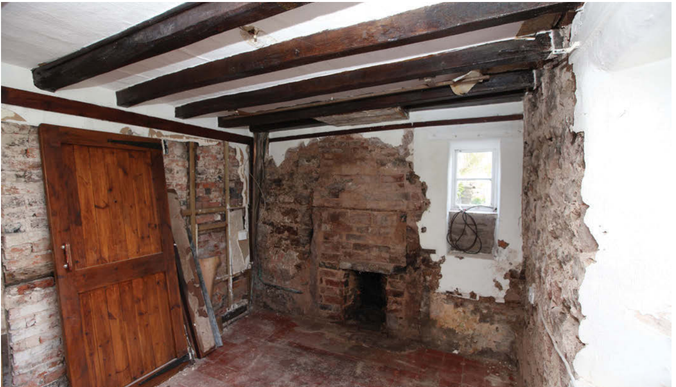
Pl. 7 Detail of parlour wall with blocked up fireplace. The adaptation of this room into a kitchen will require new plumbing, sink waste and services will be located on the fireplace wall. Lime plaster will be reinstated to the fireplace wall and front wall, in combination with kitchen fittings which are slightly off-set from the damp walls.
