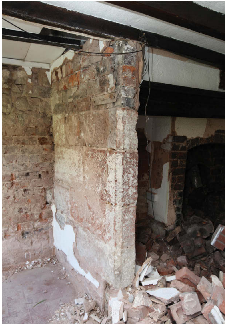
Pl. 6 (right) the Artex and gypsum plaster has been removed to reveal the ashlar heck screen stub wall, with dressed pink gritstone. Brickwork above the screen and along the gable wall of the lobby will be finished in lime plaster but the ashlar will remain visible and simply brushed down.
