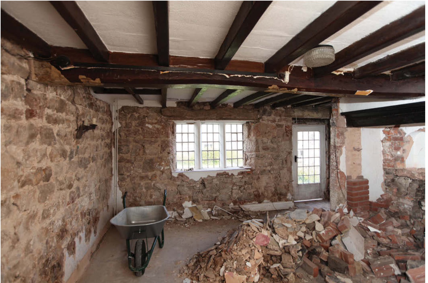
Pl. 3 View of the front wall with concrete and cement render removed. The window cill to the front window will be reinstated to its original level and the walls will be re-plastered in lime plaster.
