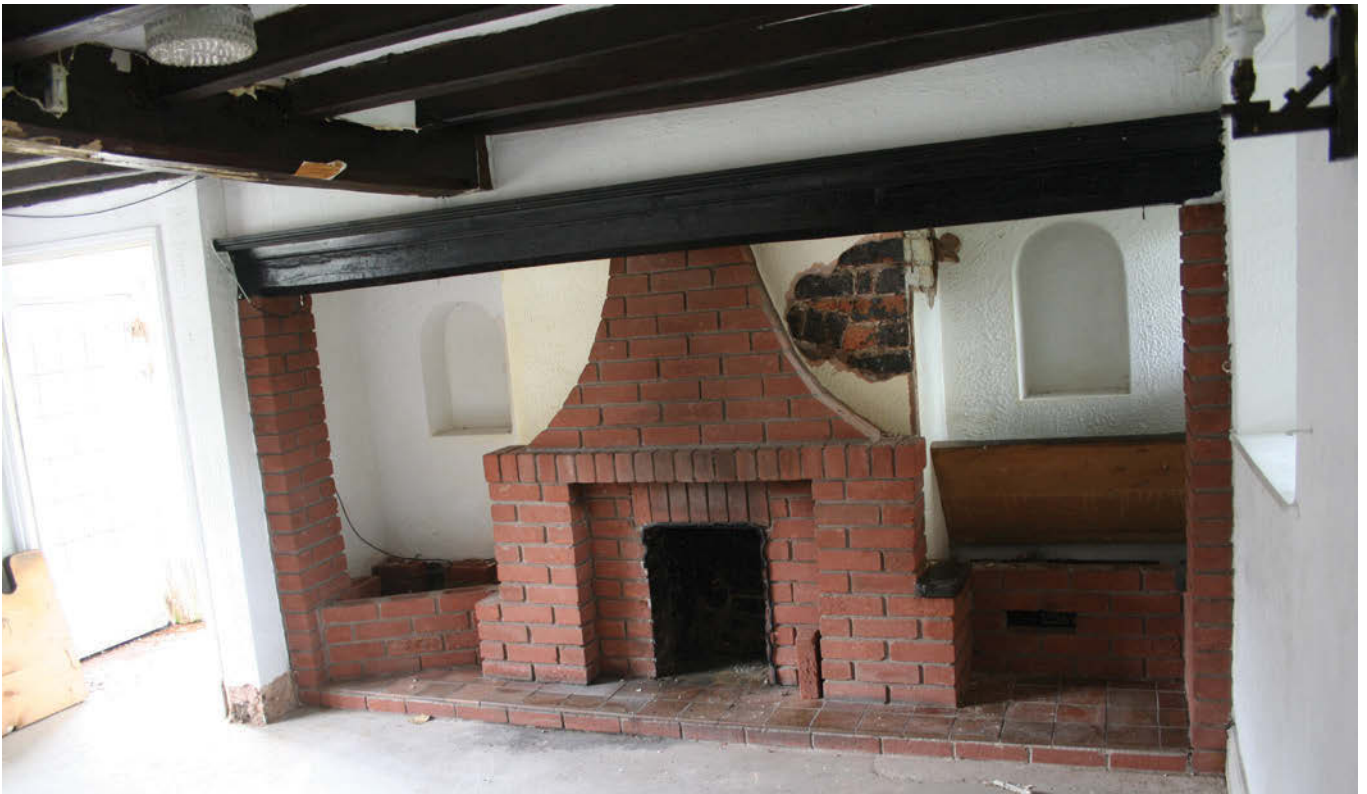
Pl. 1 Firehood to former House Place, with inserted modern brick hearth. This modern brick hearth has been removed by agreement
