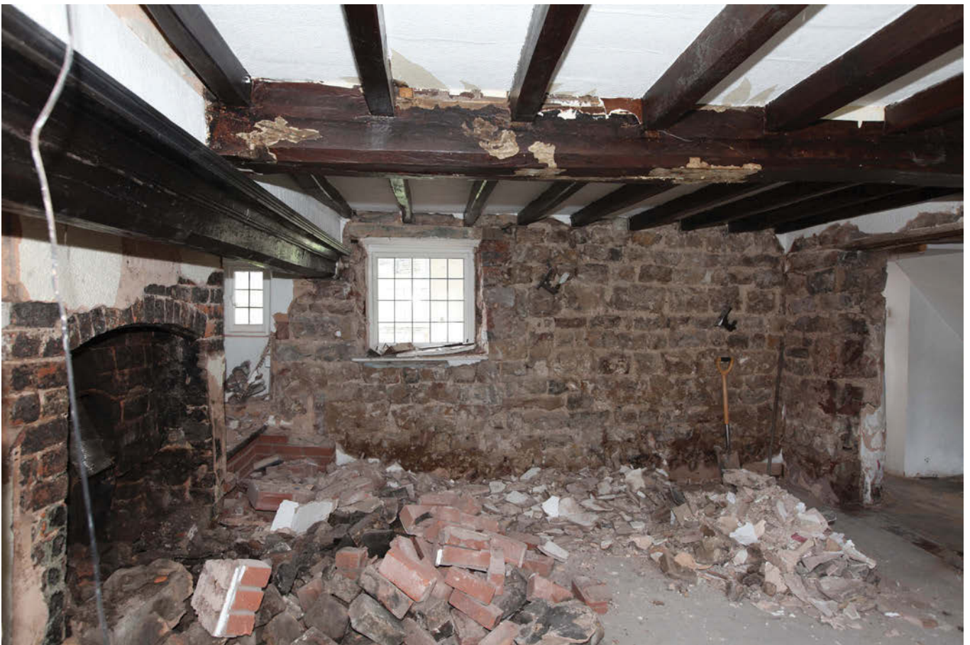
Pl. 4 Back wall to House Place, with fire window and modern leded-light. Artex and gypsum plaster has been removed and the wall is drying out. The proposals involve replacing the rear 'mock-leaded' window with a new pair of side-hung timber casements with single horizontal glazing bar.
