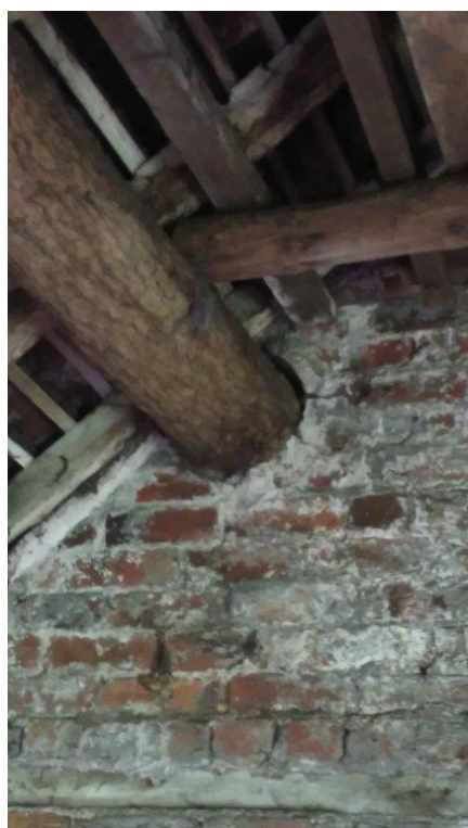
Plate 4: Crevice in brickwork where beam enters wall in pig shed
