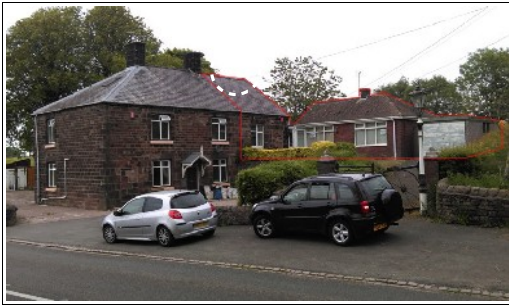
Figure 4. West elevation (outlined red) *Ingress points around roof section (White dashed)
