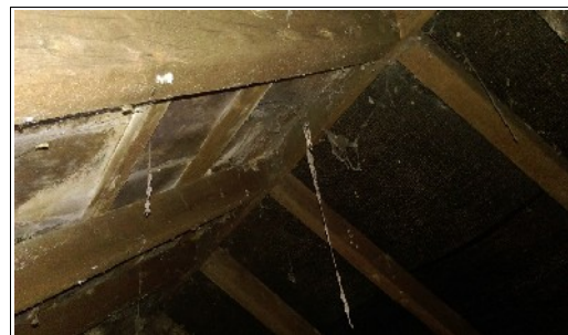
Figure 10. Roof part plaster torching and underfelt.
