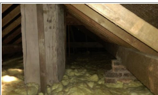
Figure 11. Apex roof void above bungalow.
