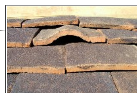
Fig.14. Examples of bat access tiles and soffit slits
