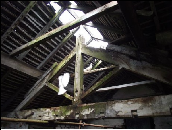
Fig.8. Roosting pigeons + broken roof section in the single-storey, central connecting section.
