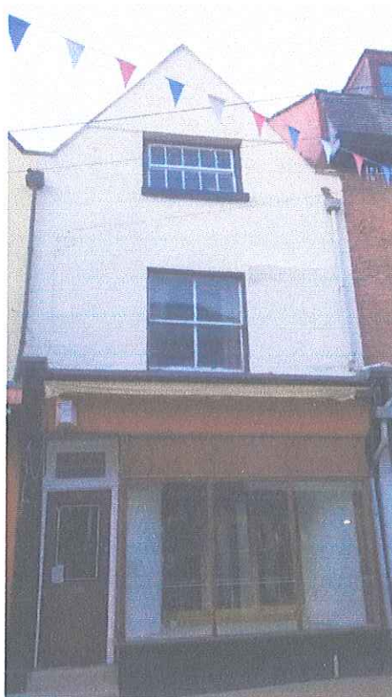
General View of the Front Elevation of the Existing Building
