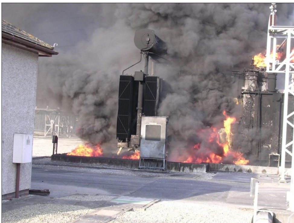
Figure 6: Catastrophic Failure at a Primary Substation
