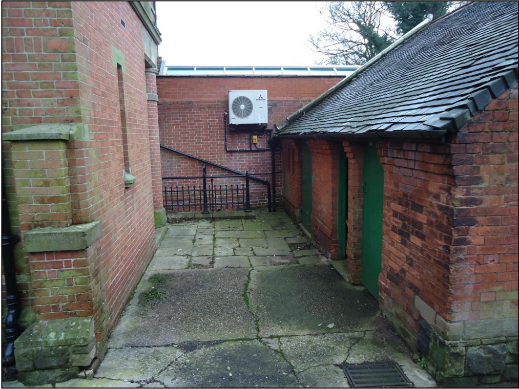
Photograph 4 . Area to receive proposed walkway from existing building to proposed extension
