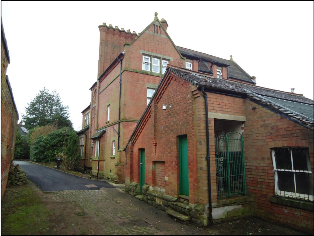
Photograph 3 . Hard standing area to have proposed additional parking space
