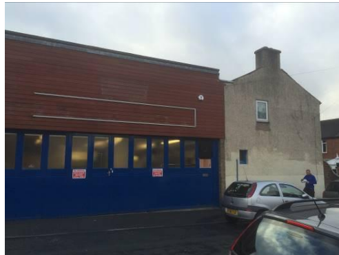
No.82 adjoined to laundrette building
