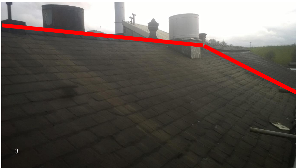
3. Part of the slate tile roof (red box) to be replaced looking South at the western aspect.
