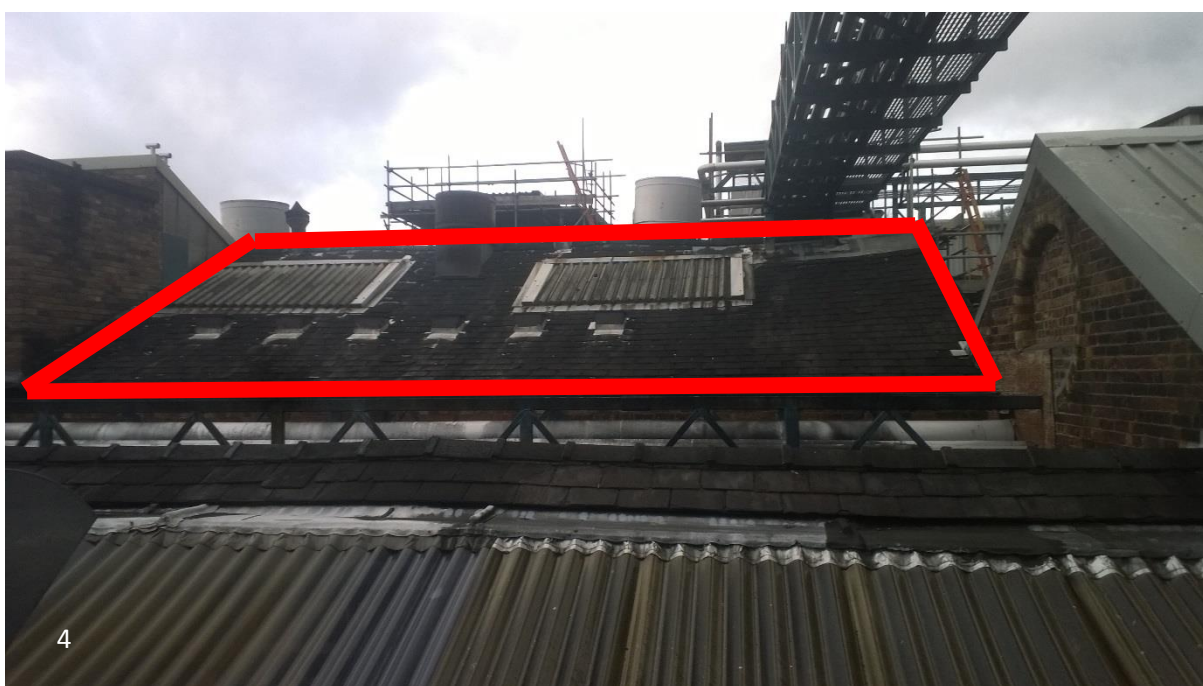
4. Part of the slate tile roof (red box) to be replaced looking West at the eastern aspect.
