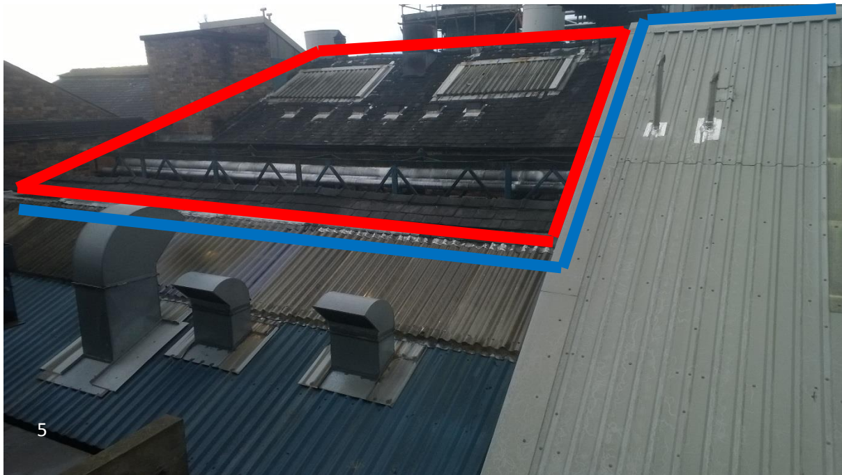
5. Part of the slate tile roof (red box) to be replaced looking West at the eastern aspect and 2 adjacent roof (blue box) materials for comparison.
