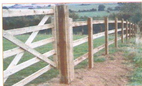
Post and rail. 4" X 2" rails on 6" X 3" posts alongside a medium weight five bar field gate. All posts have weathered tops.
