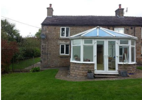
Fig.5 South Elevation indicating existing conservatory. Conservatory does not provide all year round space or enough of a connection to the external garden Materials: UPVC with stone plinth
