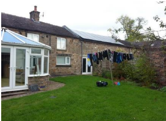
Fig.5 South Elevation indicating existing conservatory. Conservatory does not provide all year round space or enough of a connection to the external garden Materials: UPVC with stone plinth
