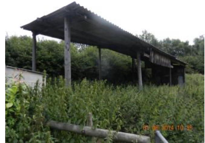
Existing Hay Store Structure - South Elevation
