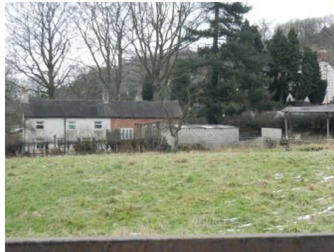
Existing Barns - Blockwork Store - South Elevation
