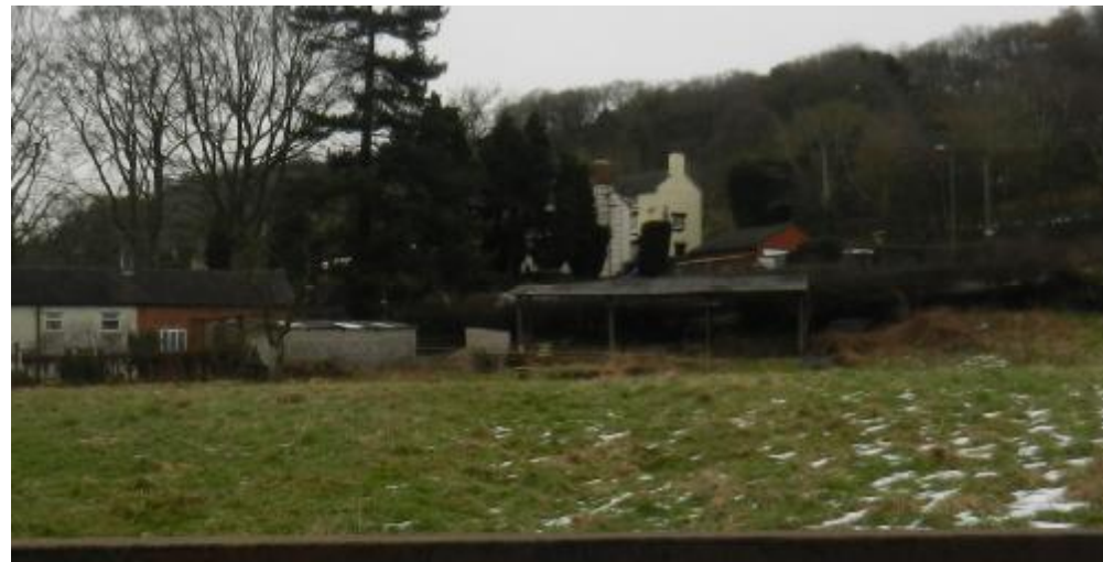
Existing Hay Store Structure - South Elevation - From the Site Boundary
