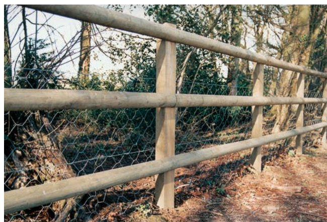
Post and Rail fencing (nailed) with half round rails
