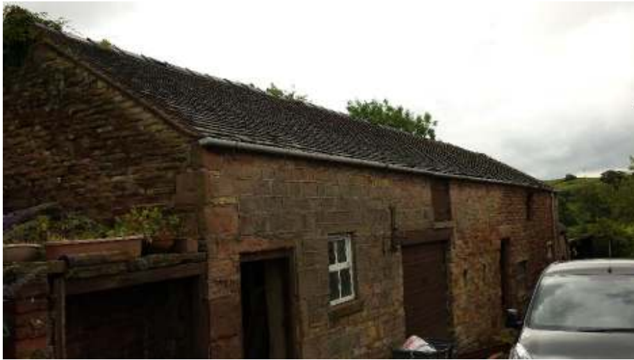
Plate 1: Showing main section of the barn
