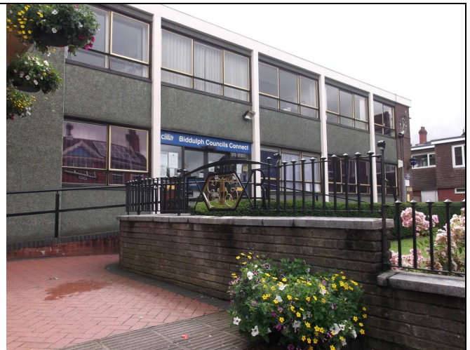
02: Existing elevation with columns and rendered panels.
