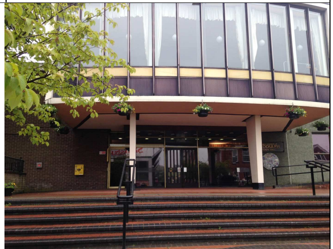
04: Stepped approach to where main entrance will be.
