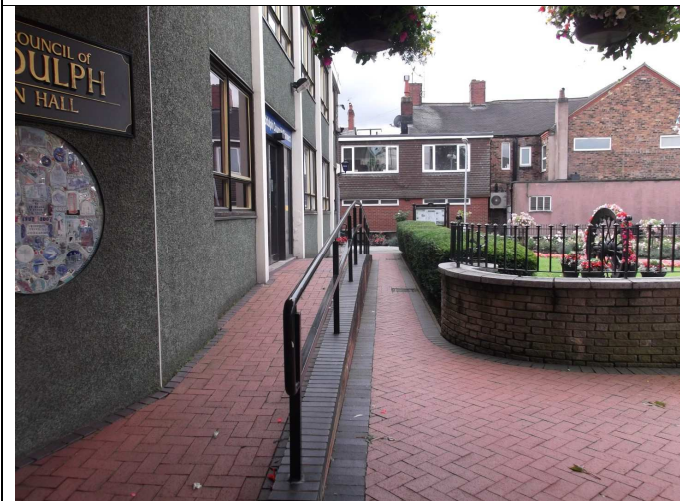
03: View of ramp to be removed and approach widened.
