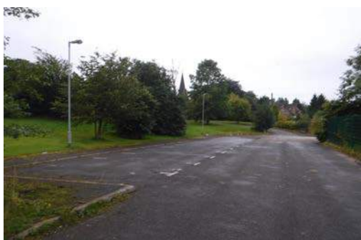
View south across former car park, with landscaped area to the east
