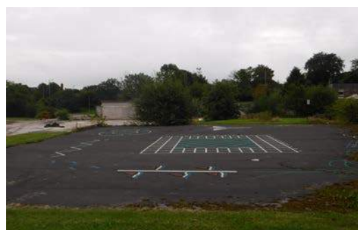
View east across former playground, with existing floor slab to the north
