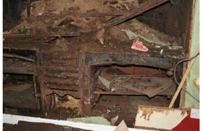
Details of the cast-iron range: Above - double ovens. Below left - chimney flue with iron bands lining large circular flue. Below centre - the wall to the rear of the former doorway, with straight joints. Below right - collapsed plate warming rack
