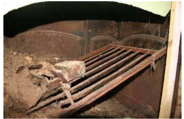
Details of the cast-iron range: Above - double ovens. Below left - chimney flue with iron bands lining large circular flue. Below centre - the wall to the rear of the former doorway, with straight joints. Below right - collapsed plate warming rack
