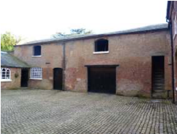
Plate 1: Showing building B that was surveyed.
