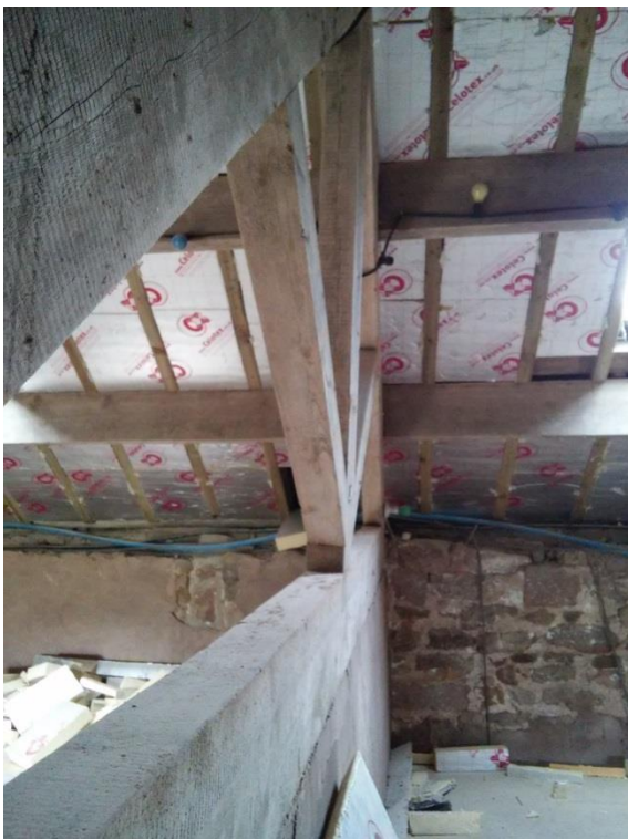
Two of the main kingpost trusses have distorted out of plane. This probably occurred during a period when the roof was in a poor state of repair such that the degree of lateral restraint was inadequate, and the moisture content of the timbers was high due to ingress of rainwater. This is not of serious structural concern.
