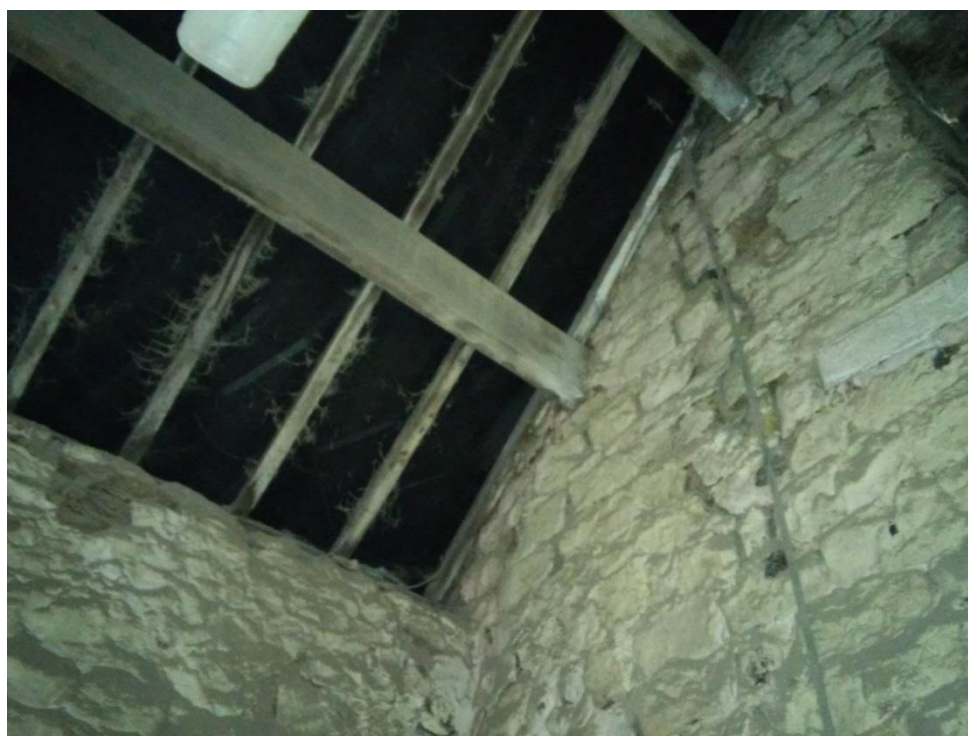
Evidence of splitting of the end gable wall at the southeast corner at high level between the purlins
