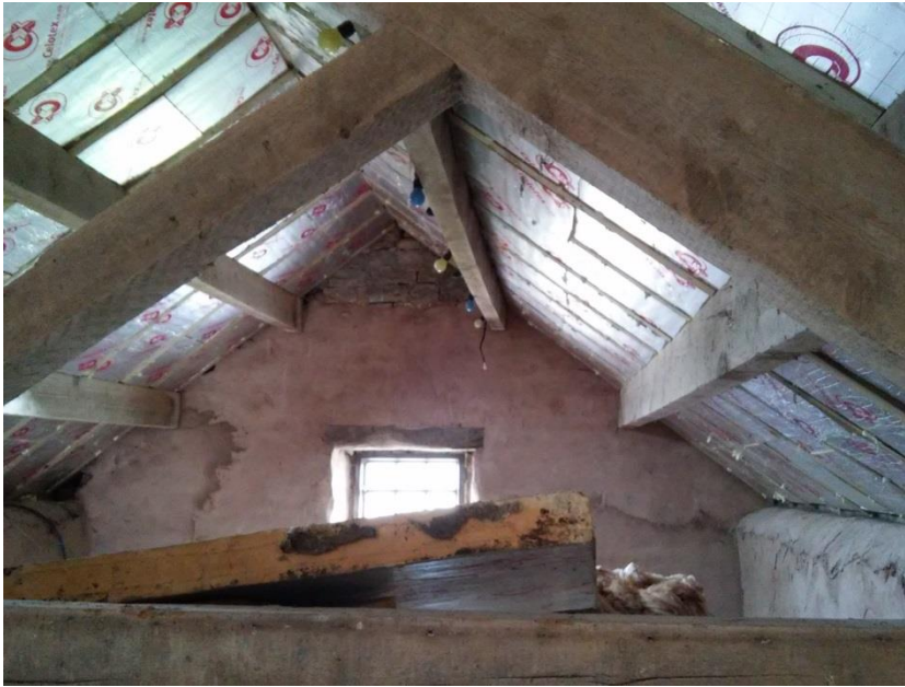
Typical roof arrangement which is very traditional but does result in outward thrusts being applied to the tops of the main sidewalls
