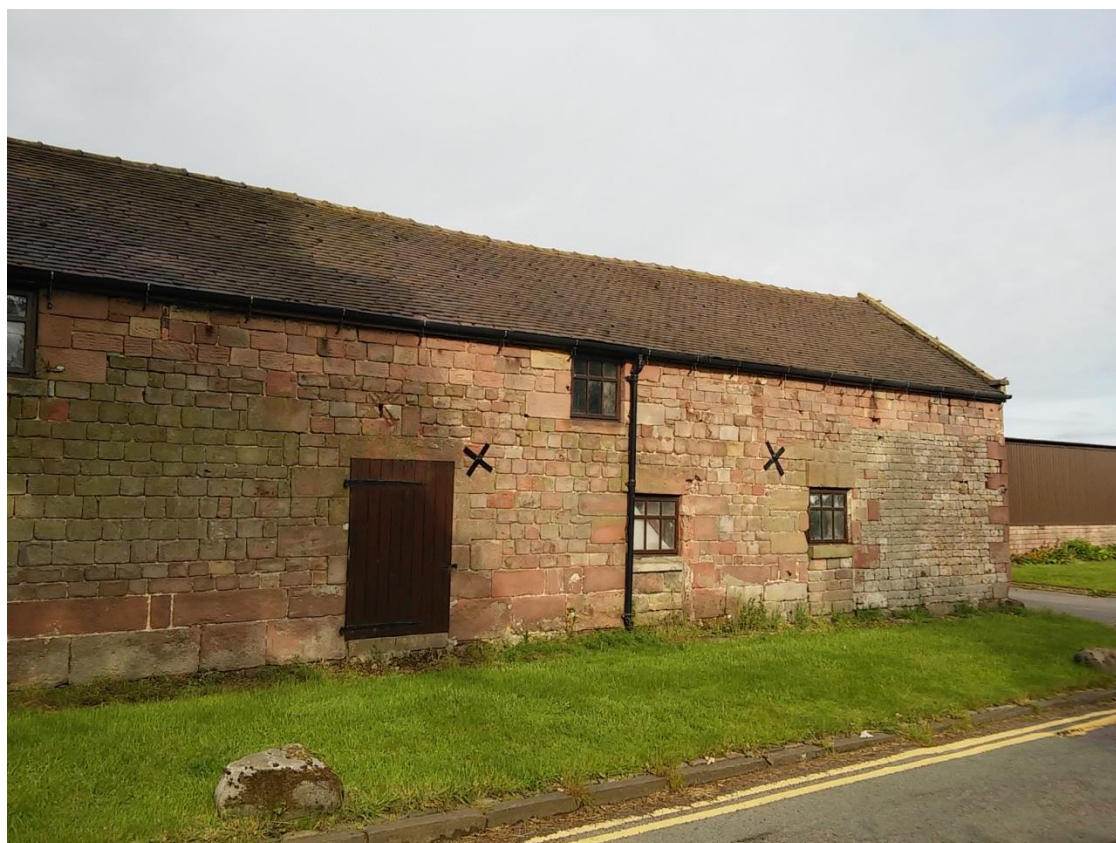
Partial View of Main East Wall – note coursing appears quite regular without excessive vertical distortions
