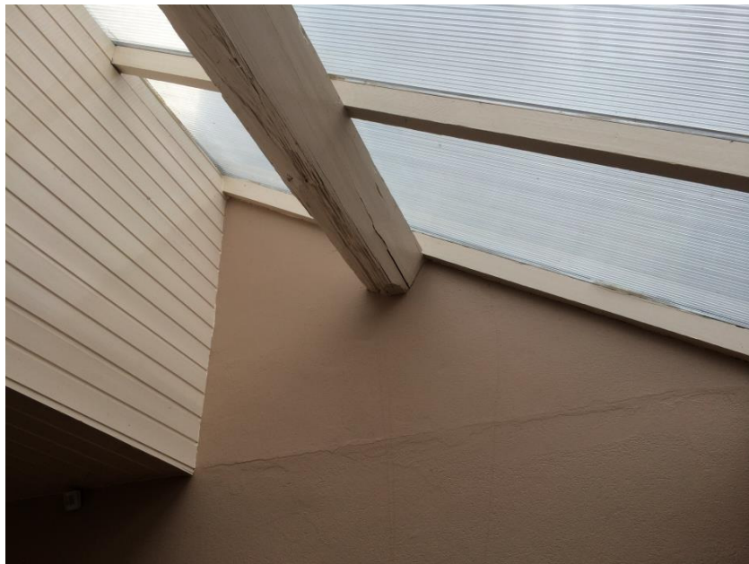
Photograph 7 – Splitting of timber purlin
