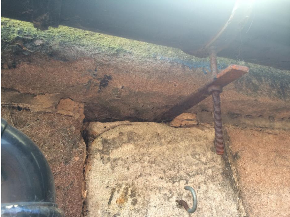
Photograph 9 – Loose gutter brackets
